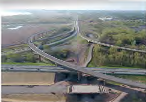
An aerial view of the I-41/I-43 interchange, looking east at I-43.
