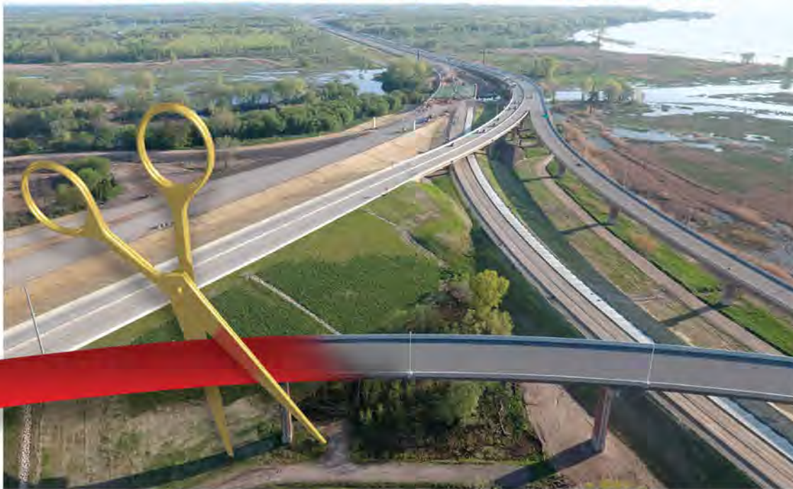
The I-41/I-43 interchange, spring 2016.
