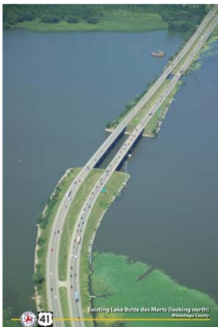
Existing causeway looking north
